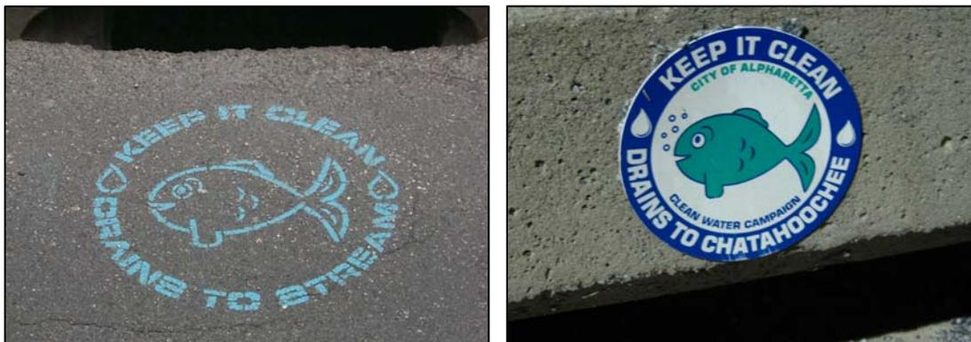
**Figure 2-3 Example of a Stormwater Drain Stencil and Curb Marker**
