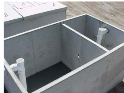
Figure 3. Multi-compartment septic tank
