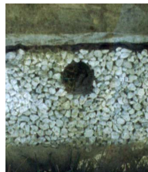
Figure 4. Gravel filled trench
