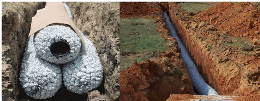
Figure 6. Absorption trenches containing bundles of polystyrene aggregate in place of gravel.
