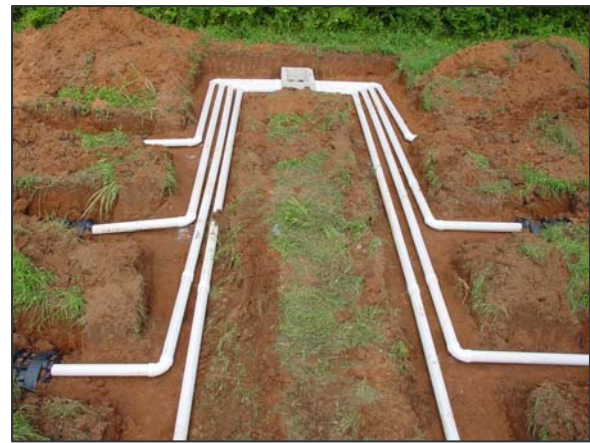
Figure 8. Distribution Box Absorption Field Design
