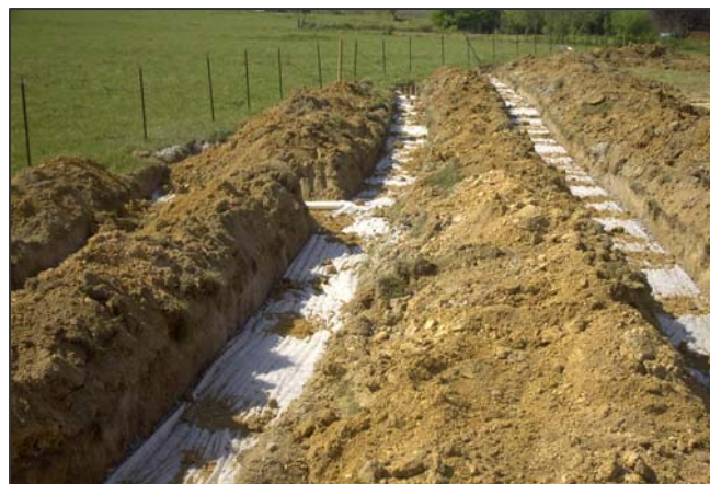
Figure 9. Serial Distribution Absorption Field
