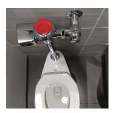
\*A flush volume may be listed on the porcelain of the toilet. Ignore this number because the flush valve is what determines the flush volume.
