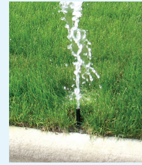
Improperly functioning rotor sprinkler head
