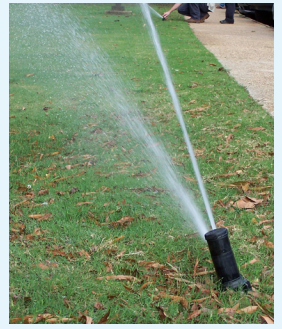
Improperly functioning rotor sprinkler head
