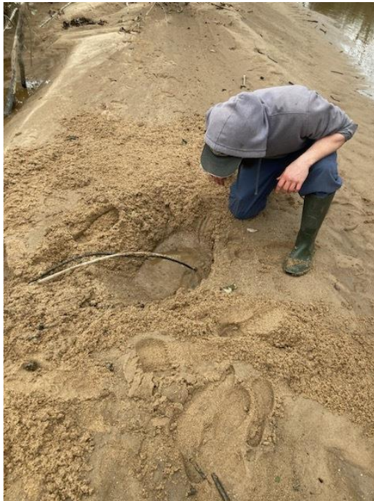
West Fork, buried intake after storm moved sediment.
