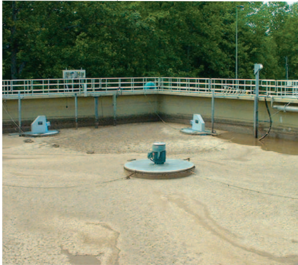
Sequencing Batch Reactor
