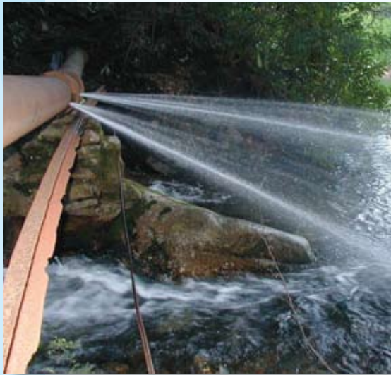
Fixing leaks can lead to both water and financial savings.
