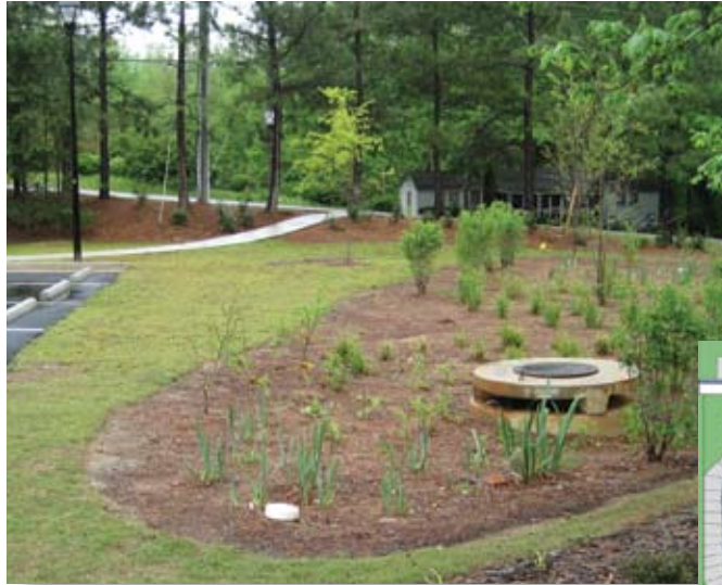
Rain gardens treat stormwater and provide drought-resistant landscaping in the City of Alpharetta.
